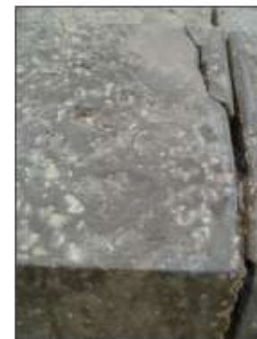
Photo 16 Repair Procedure No. 2. Replace 1/2" Expansion Joint Material.
