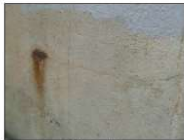
Photo 13 Repair Procedure No. 3 and No. 4
