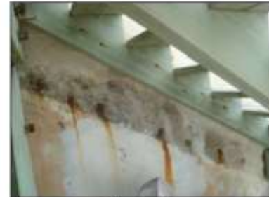
Photo 12 Repair Procedure No. 3: Cut Back Steel.
