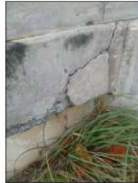
Photo 11 Repair Procedure No. 2
