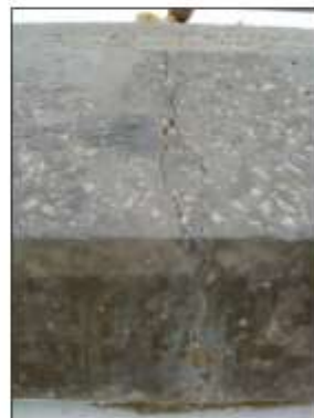
Photo 14 Repair Procedure No. 2
